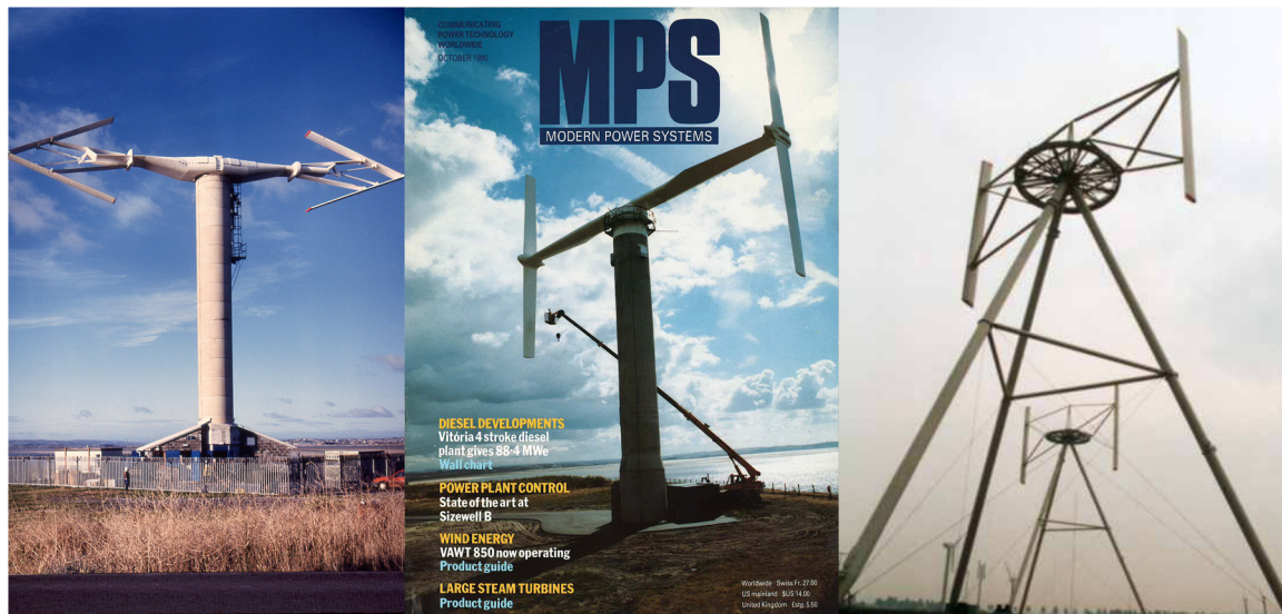
Fig. 4. Left: The 130-kW variable-geometry VAWT-450 with the blades reefed (the blades were straight at maximum power mode). Photo by Jos Beurskens. All rights reserved. Center: The 500-kW VAWT-850 as featured on the front cover of Modern Power Systems in the 1990 October issue. Used with permission from Modern Power Systems. Right: The Heidelberg 300-kW H-rotors in Kaiser-Wilhelm-Koog. Photo by, and used with permission from Jörg Bendfeld.
