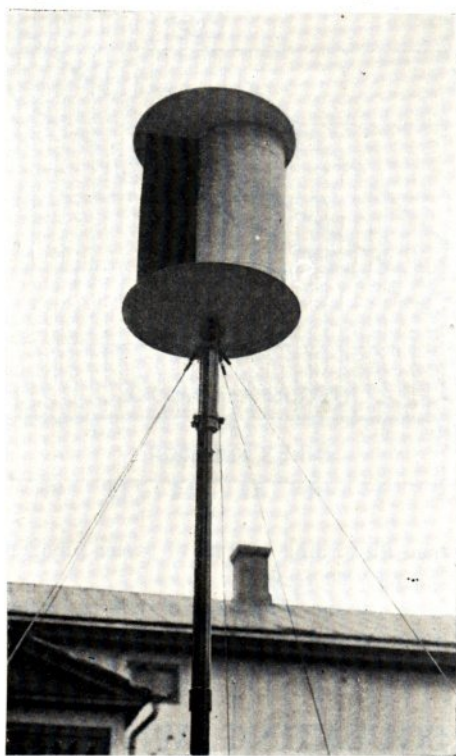
Fig. 21. A Pumping Wing-Rotor fixed to the top of a tubular mast. The two ball bearings are in the short tube clamped to the mast. The brake is situated under the lower endplate, the wire nearest the mast actuating the brake. The other four wires are stays.
