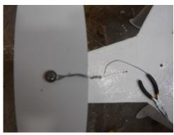
Step 6. You can cut blade tips from thin plywood or plastic. Use silicone caulk and 3/4" long #8 wood screws with washers to attach onto blade ends.
