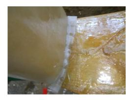
After the first coat dries for a couple hours, use a high speed rotary sander with 100 grit and sand down high spots and loose bits.
